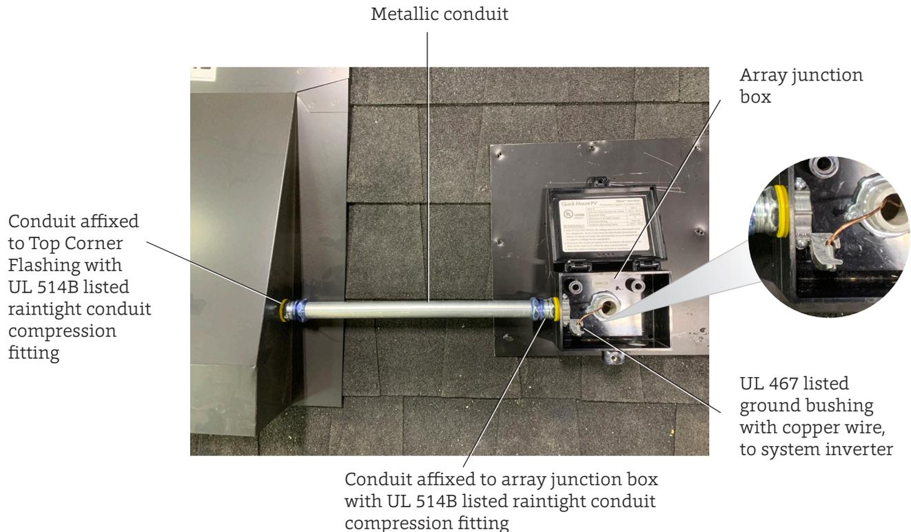
**Figure 11. System grounding**
