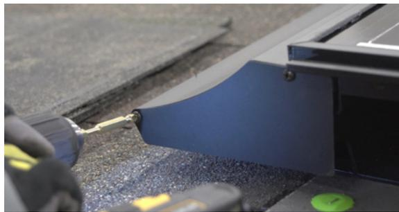
**Figure 50. Install Starter Bar covers**
