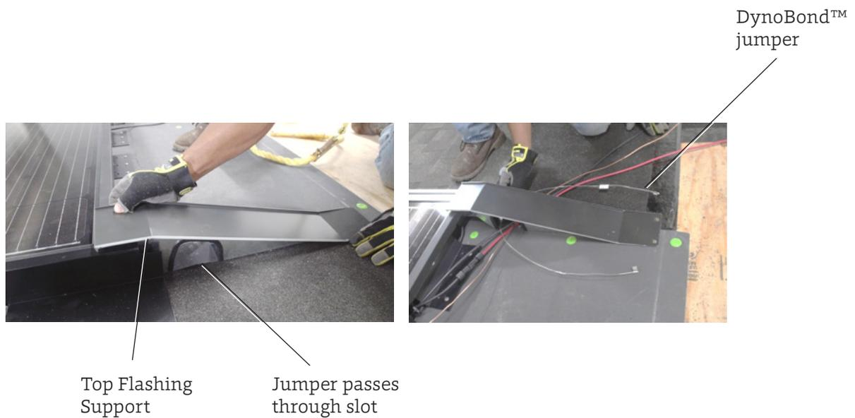
**Figure 10. DynoBond™ clip connection, module frame to Debris Guard**
