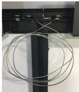
**Figure 44. Installing DynoBond<sup>™</sup> Jumpers between modules**
