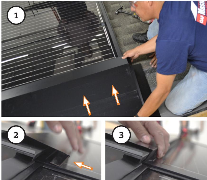
**Figure 58. Position the Top Flashing**
