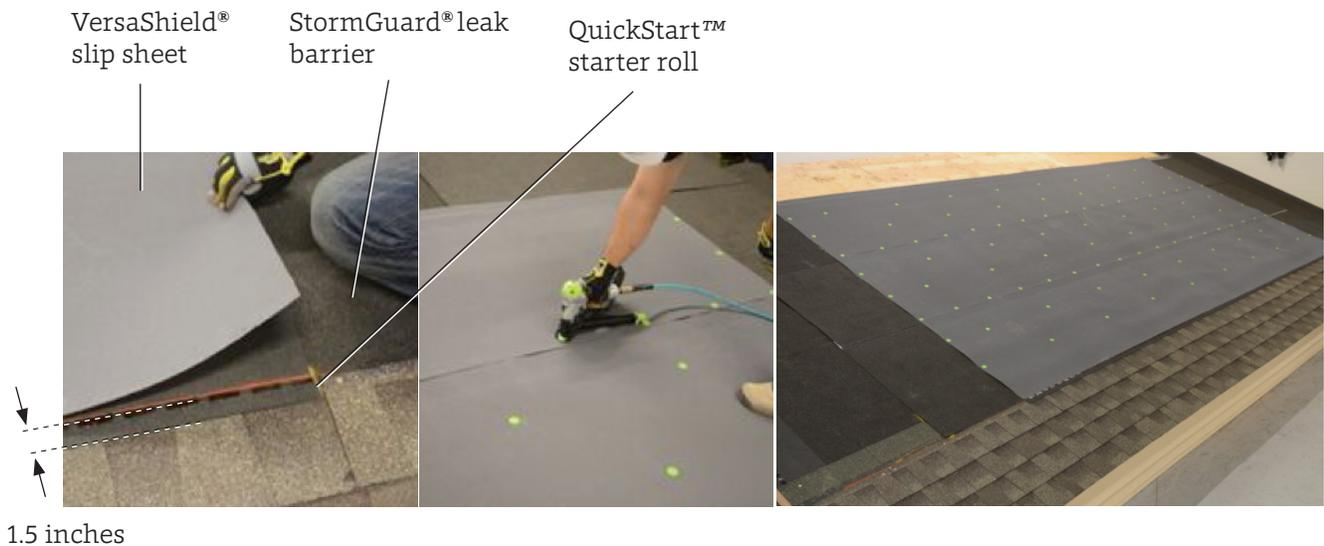
**Figure 23. VersaShield® roof example**
