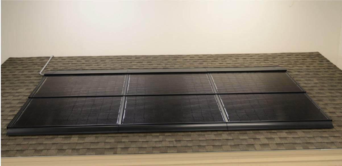
**Figure 69. Completed GAF Energy Solar System**
