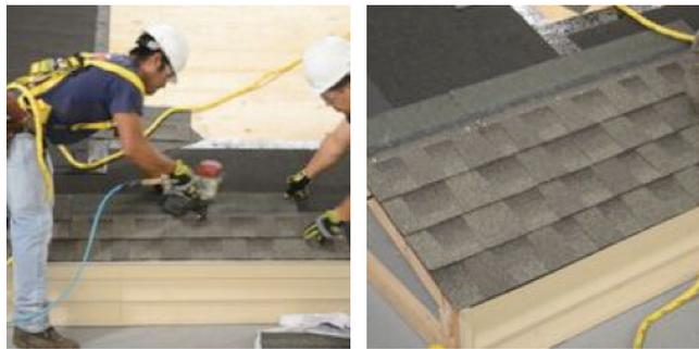
**Figure 15. Install initial rows of shingles**
