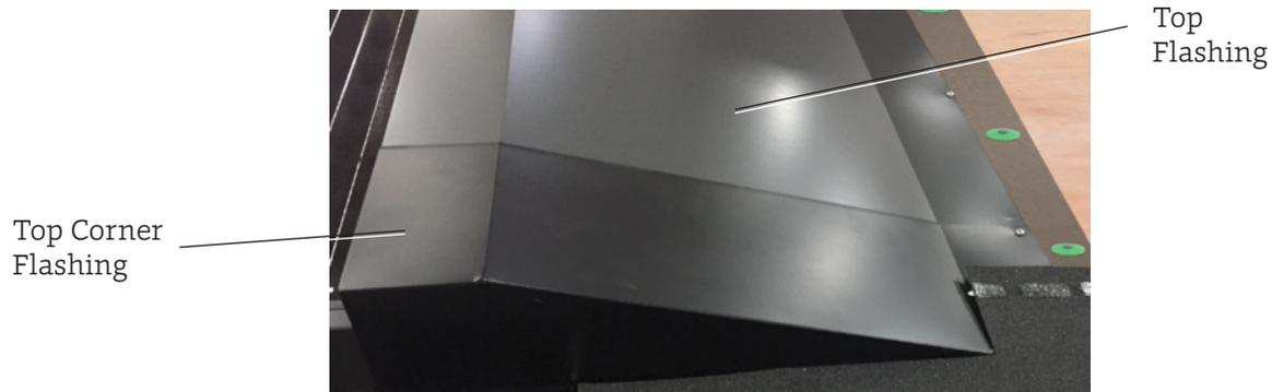
**Figure 61. Installing the Top Corner Flashing**
