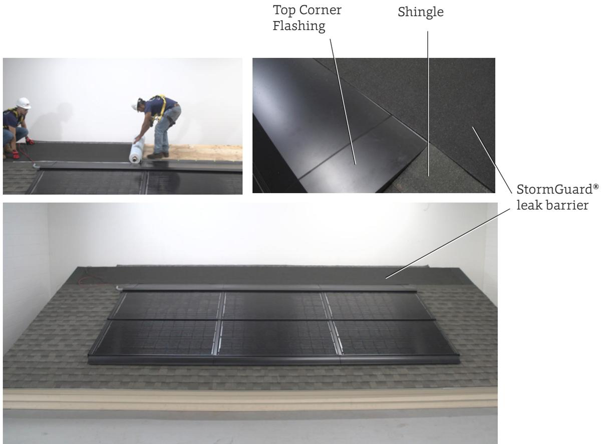
**Figure 66. Install StormGuard® leak barrier over Top Flashing and shingles**
