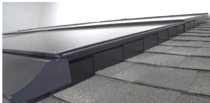
**Figure 51. Completed Step Flashing**
