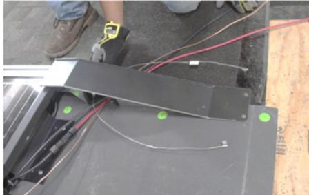
**Figure 57. Position DynoBond™ jumpers**
