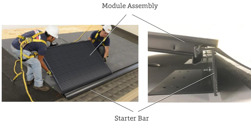
**Figure 39. Mount Solar Module Assembly onto the Starter Bar**
