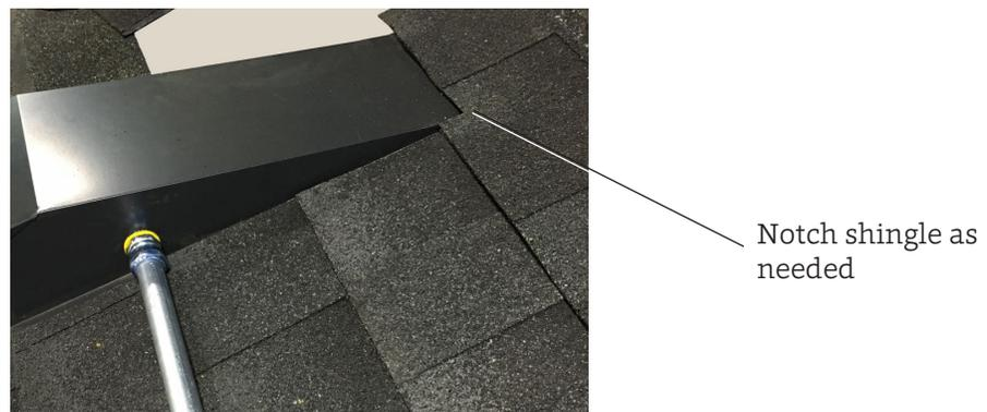
**Figure 65. Install shingles over Top Corner Flashing**
