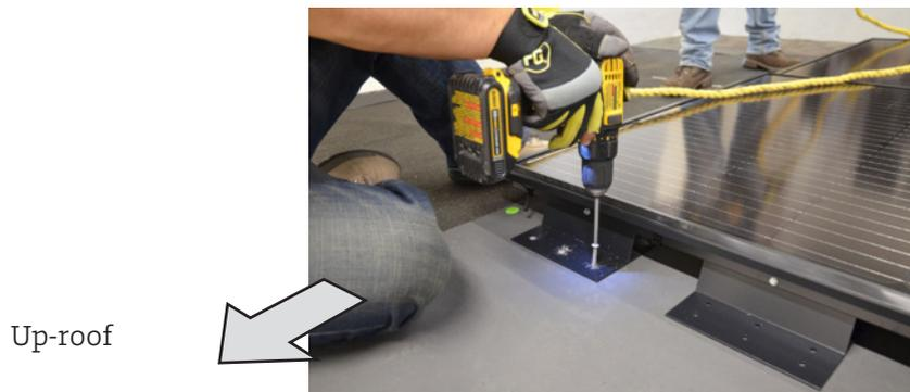
**Figure 48. Attach Solar Module Assemblies to roof deck**
