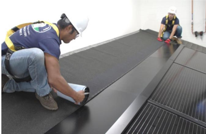
**Figure 67. Install QuickStart® over the StormGuard® leak barrier**
