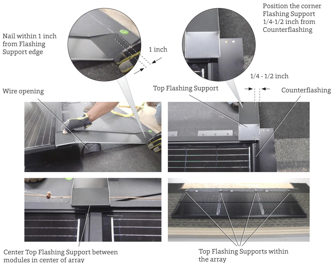
**Figure 56. Locating and installing the Top Flashing Supports**
