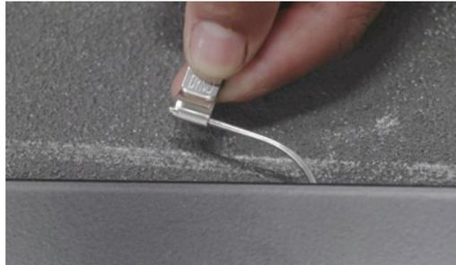
**Figure 59. Attaching the DynoBond™ grounding jumper clip to Top Flashing**
