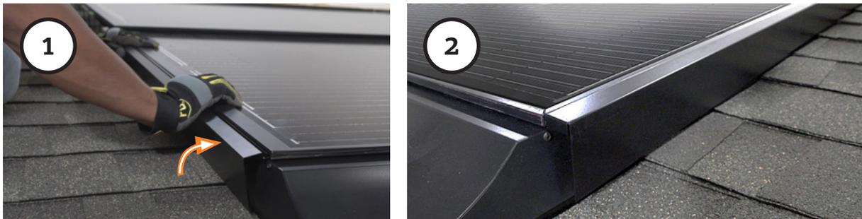
**Figure 54. Install Counterflashing**
