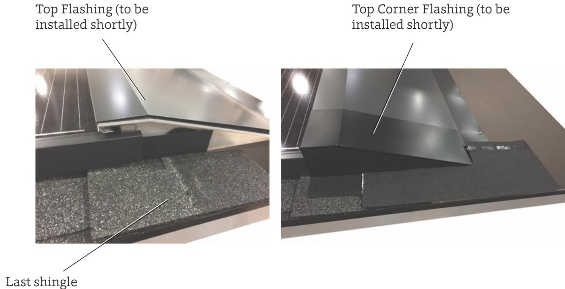
**Figure 53. Step Flashing and shingle overlap with Top Corner Flashing**
