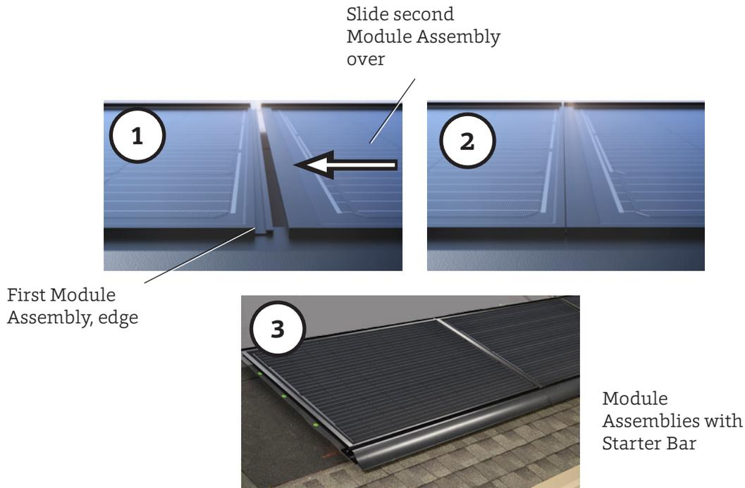
**Figure 40. Placing and aligning Solar Module Assemblies**
