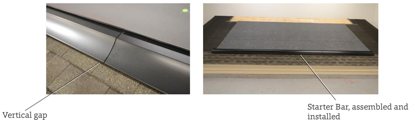
**Figure 38. Starter Bar installed on a roof**
