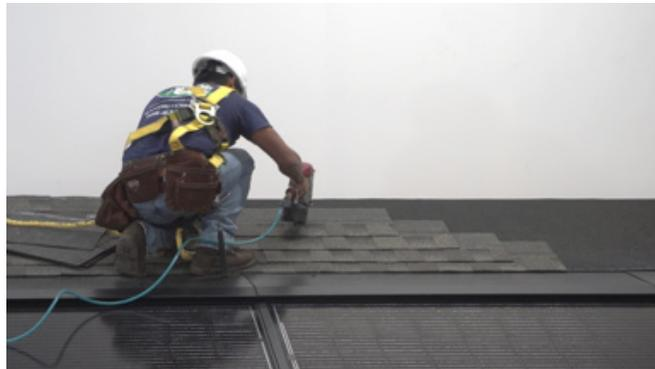
**Figure 68. Install remaining shingles and finish roof**
