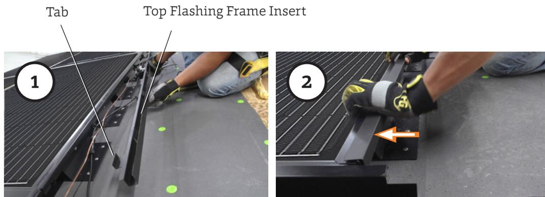
**Figure 55. Install Top Flashing Frame Insert**
