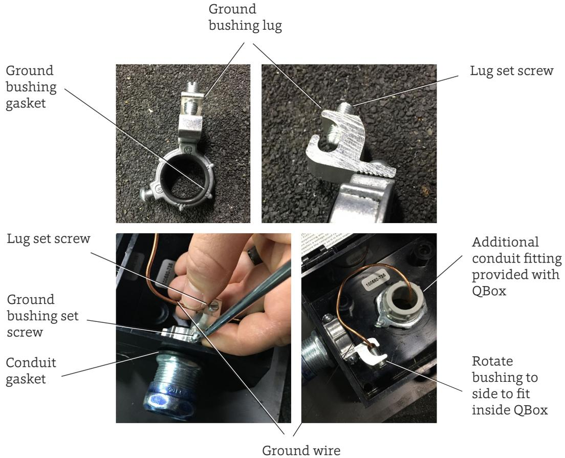
**Figure 70. Connect home runs and ground conductor to QBox**
