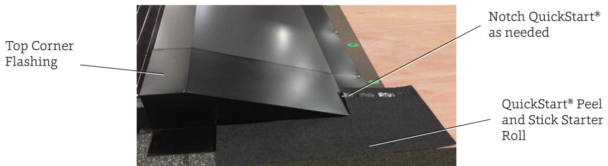
**Figure 64. Apply QuickStart® Starter Roll over Top Corner Flashing**
