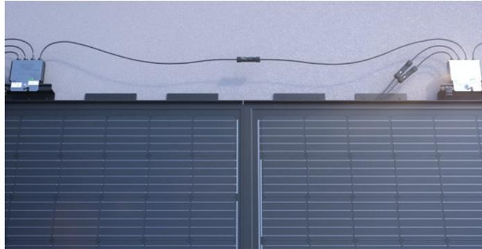
**Figure 43. Typical module-to-module connections**
