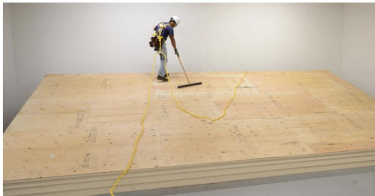
**Figure 14. Prep and clean the roof deck**
